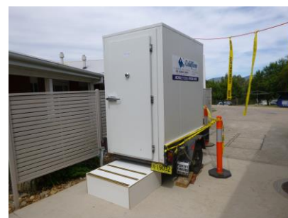
Pictured above: Freezer installation in progress
