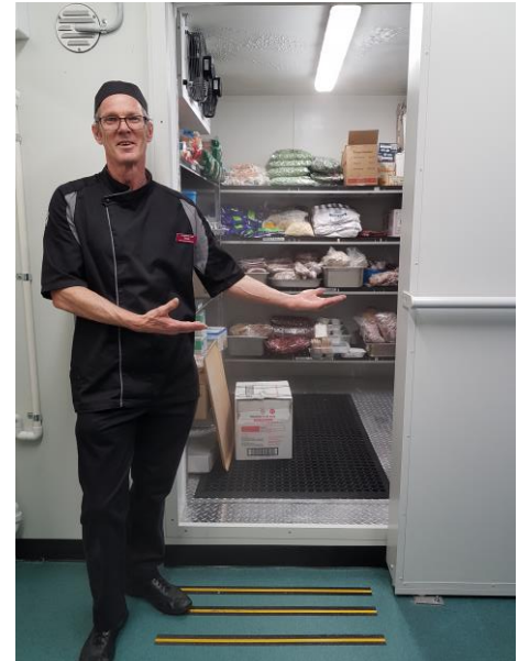
Pictured above: Our brand-new refrigerator just off the store room.
