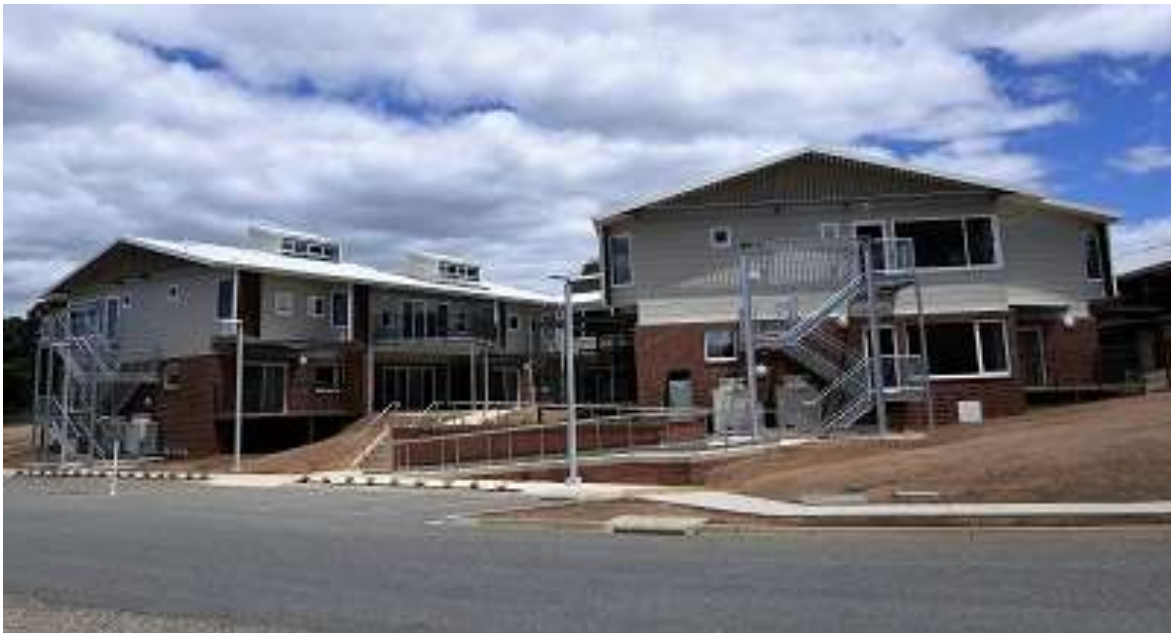
Completion of Stage One Buildings
